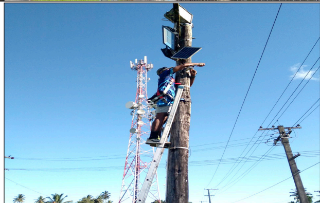
Right: Comms Staff installing CCTV Cameras at the ANZ National Stadium and the Nasinu Police Station.
